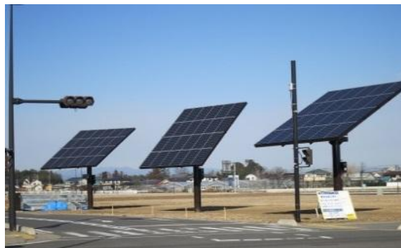
A sun-tracking solar power system (Honjo City)
