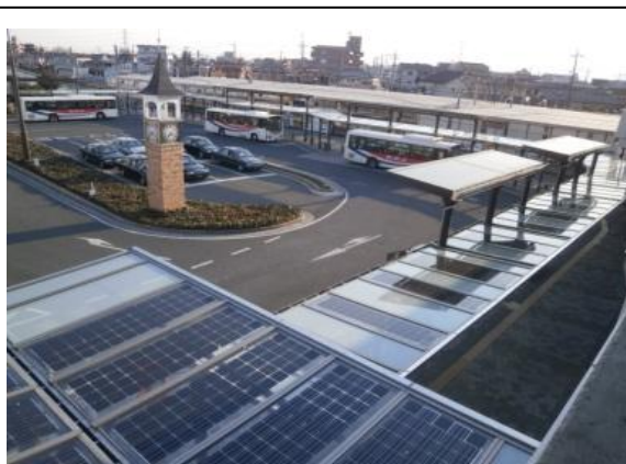
A solar power system installed in front of Tobu Railway Co.'s Higashimatsuyama Station
