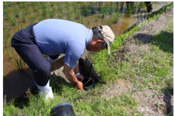
New adjustment to pipe
