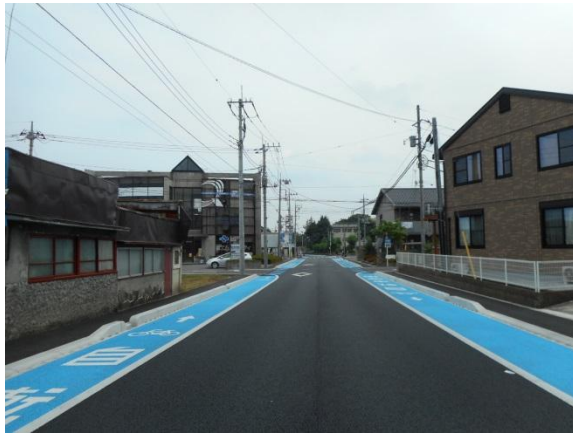
Bikeways indicated by blue surface paint on the sides of the road
