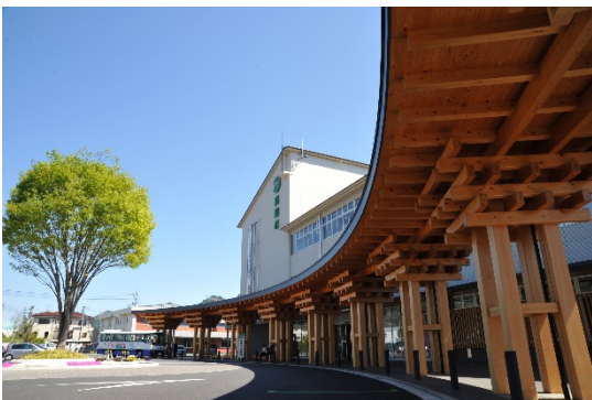
City Hall is equipped with a biomass boiler
