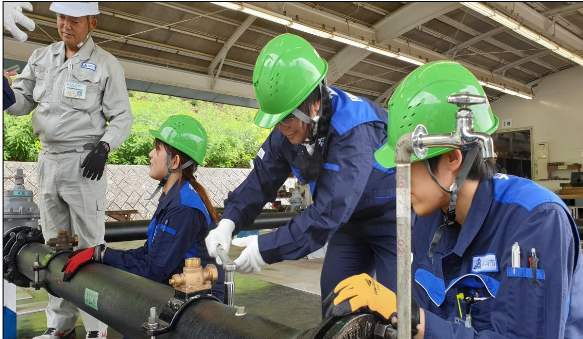
Figure 3. 150mm \Phi Ductile Iron pipe tapping work for house connection
