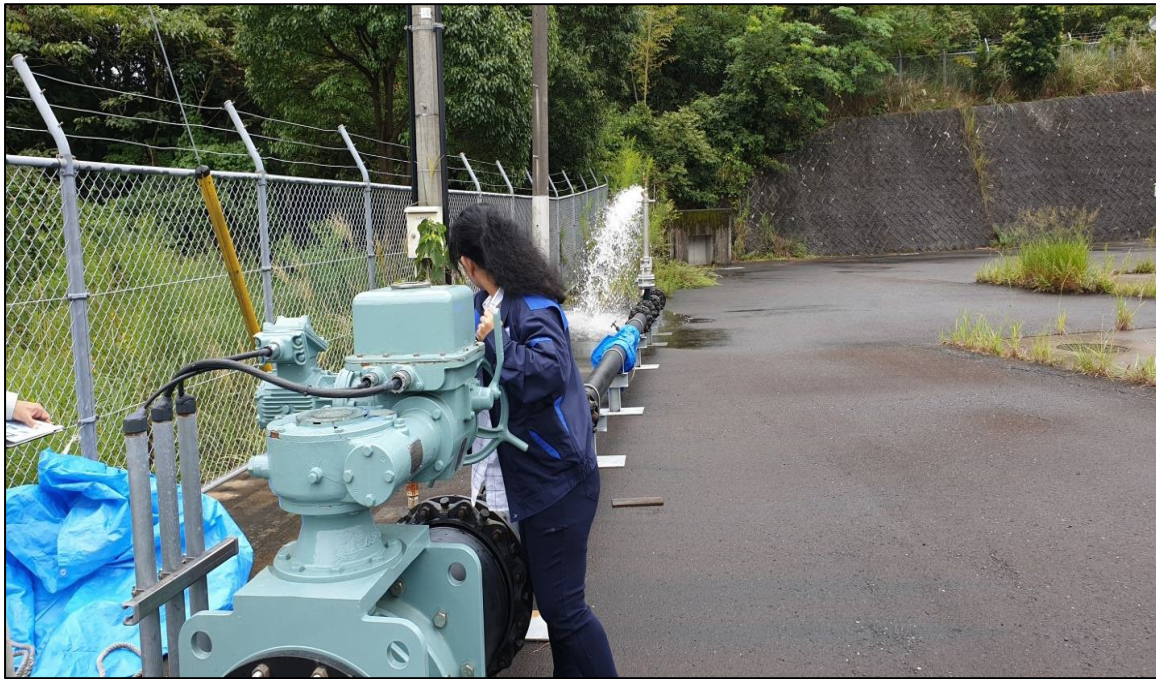
Figure 2. Electric Valve control testing
