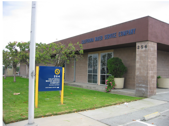
California Water Service Company, Salinas District
