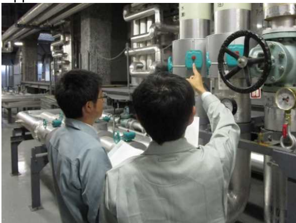
Conducting energy-saving diagnoses through plant visits
