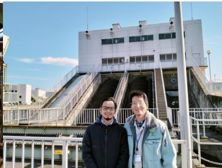
Water Pump Station
