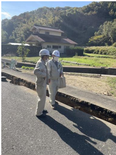
Water Pipe Replacement Site
