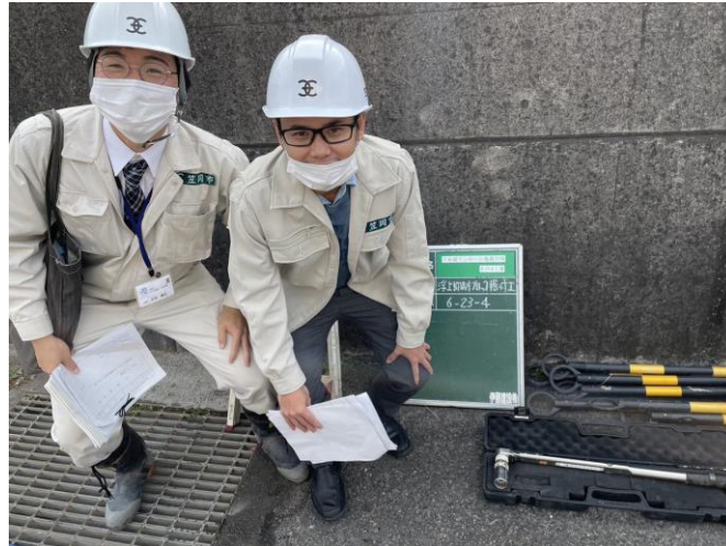
Manhole construction site
