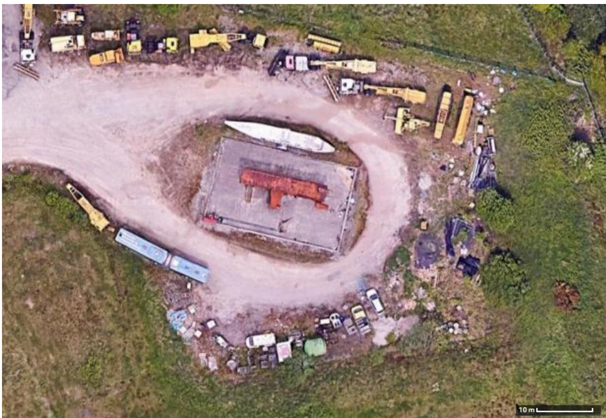
Figure 2: Fire Training Area – Leeds Bradford Airport (Google Maps, 2023)
