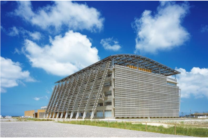
City hall equipped with a solar energy generation system on the wall and roof (Itoman City, Okinawa Prefecture)
